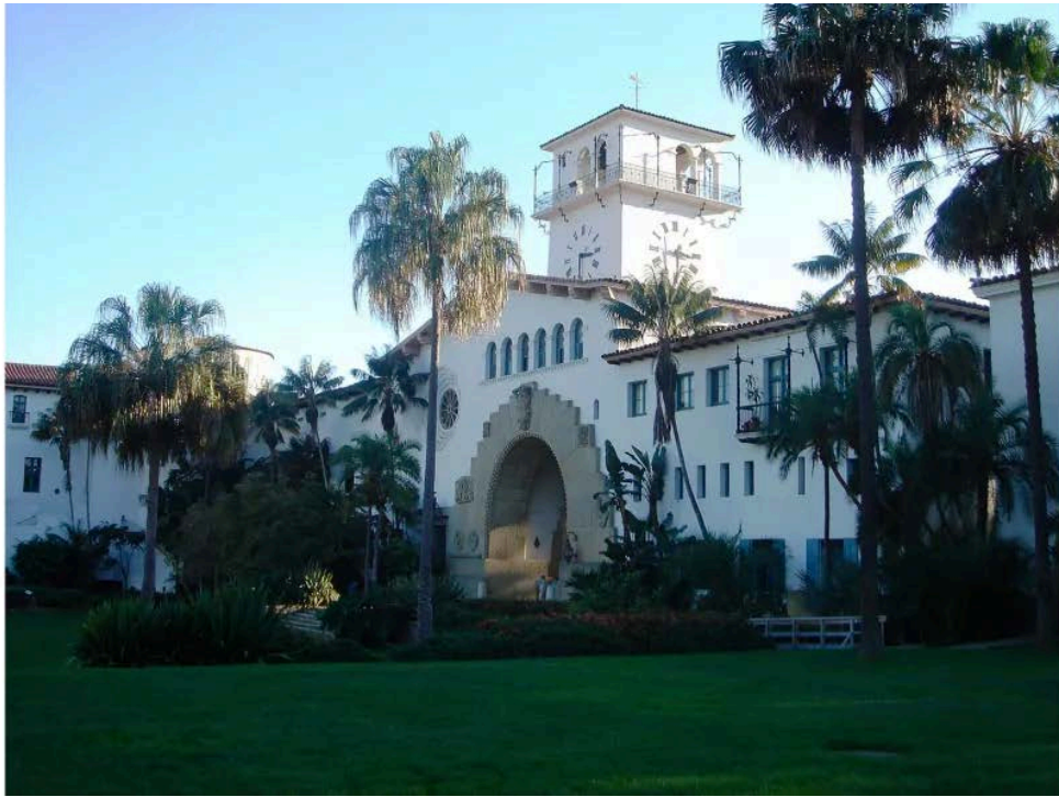
Exterior view of the Santa Barbara County Courthouse. (Public domain/via Wikimedia)
